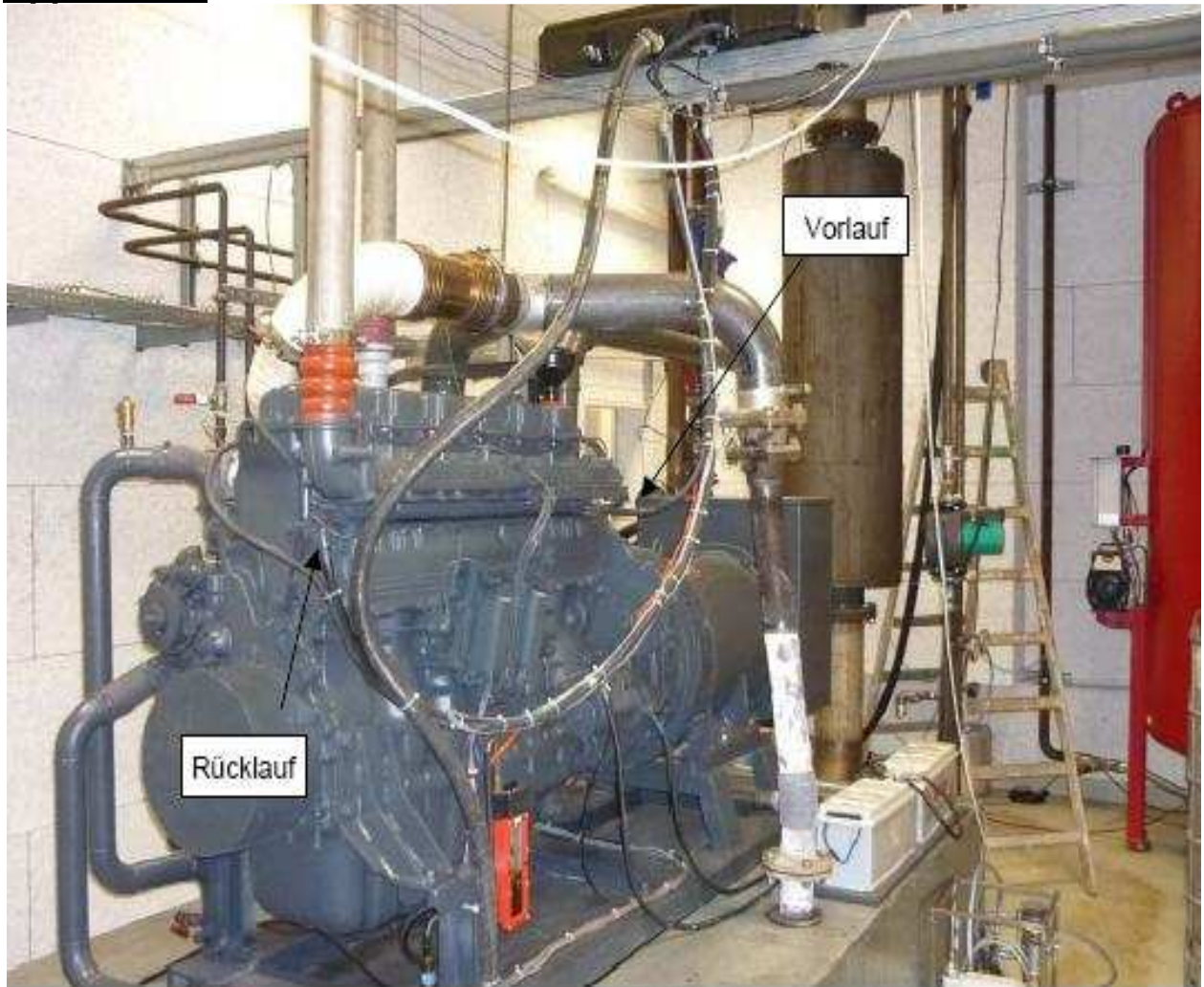
* Picture 13: View of engine with heated supply and return line.
